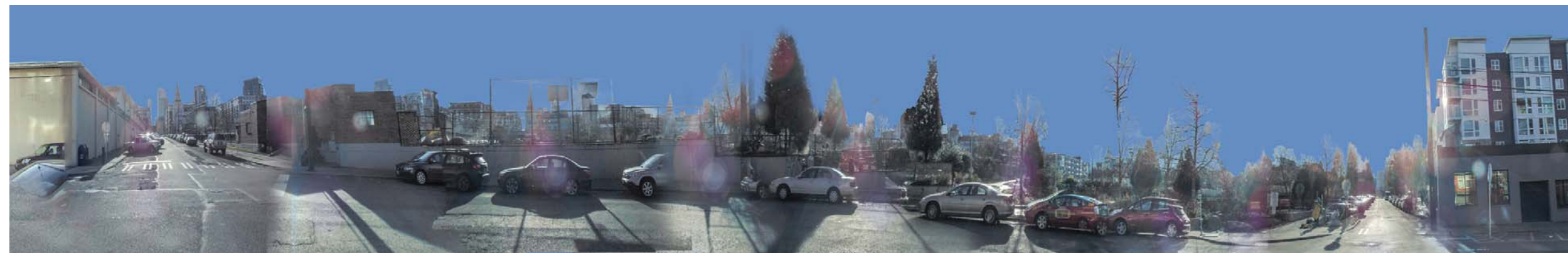
② HARRISON STREET ELEVATION, FACING SOUTH
