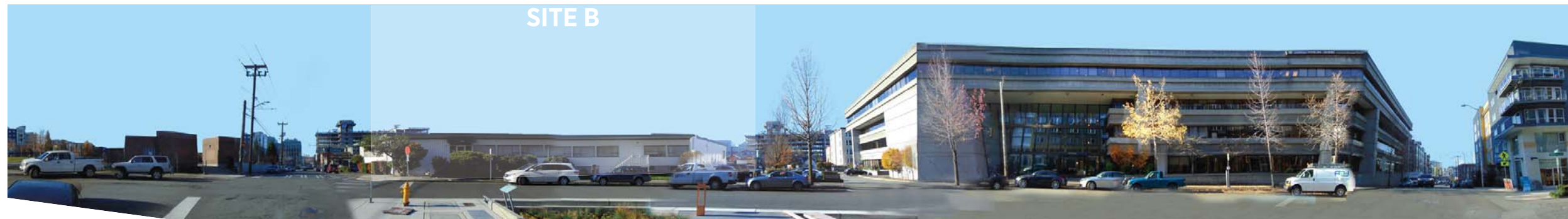
② MINOR AVENUE ELEVATION, FACING WEST
