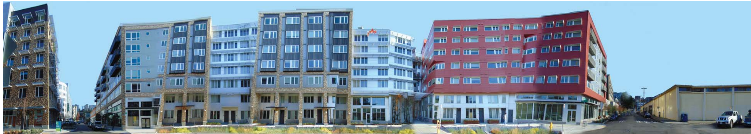
① MINOR AVENUE ELEVATION, FACING EAST
