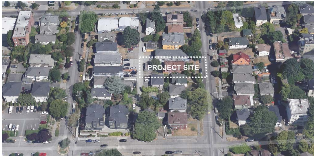
AERIAL LOOKING NORTH
