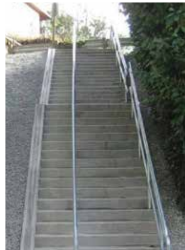
6 Staircase with Bicycle Runnel (per SDOT)
