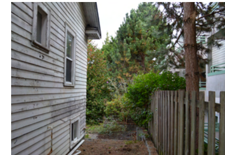
5. Looking east down property line
