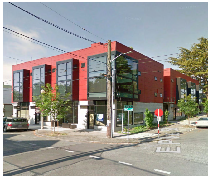
PIKE STATION LOFTS, MADRONA CONTEMPORARY DESIGN NEIGHBORHOOD APPROPRIATE
