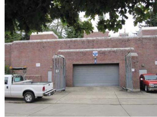
WSDOT I-90 Service Entrance
