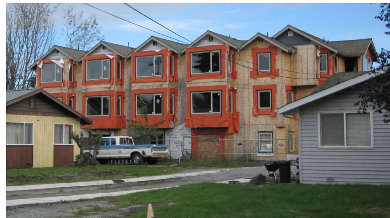
(B) Modern Design (currently under construction) across from project site
