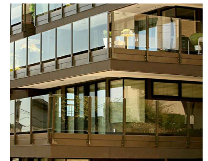
Infinity Glass Railing, Using 2" Heavy-Wall Posts with Glass Channel Welded to The Sides, and 1/2" Laminate Glass Infill
