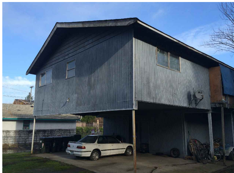
EXISTING TRI-PLEX ON SUBJECT SITE
