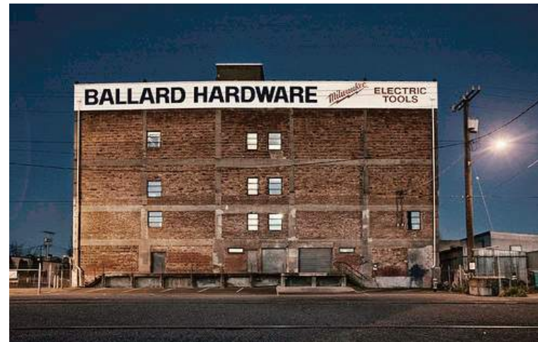
BALLARD HARDWARE - STRUCTURAL FRAME W/ INFILL
