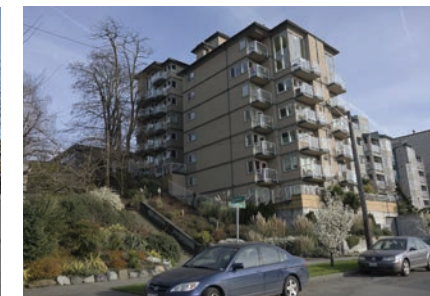
D Highmark Condominium
