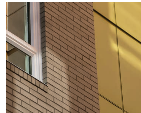
DC4 Brick and fiber cement panel contrast
