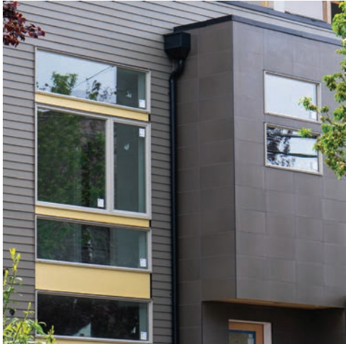
DC4 Exterior scuppers and downspouts
