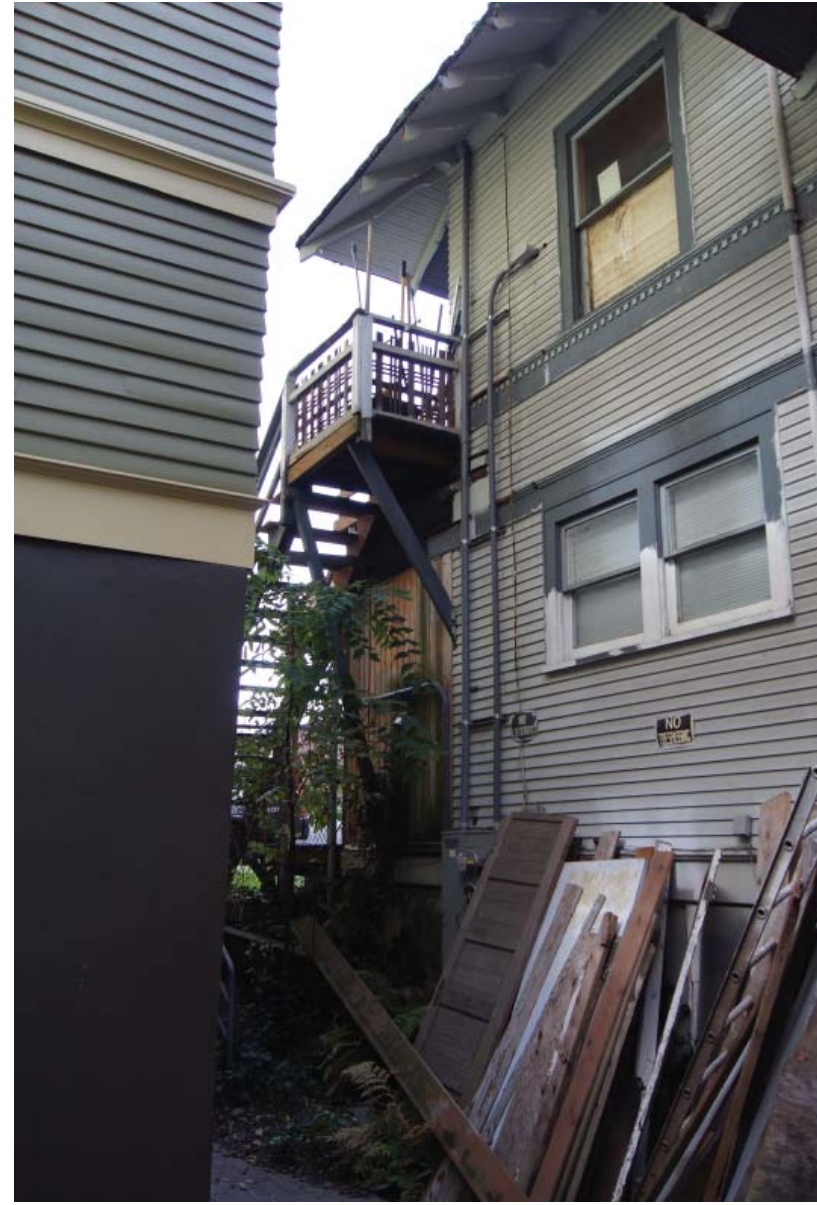
north facade of the parsonage, with the church to the left
