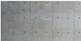
⑨ CAST-IN-PLACE CONCRETE - SNAPTIE
