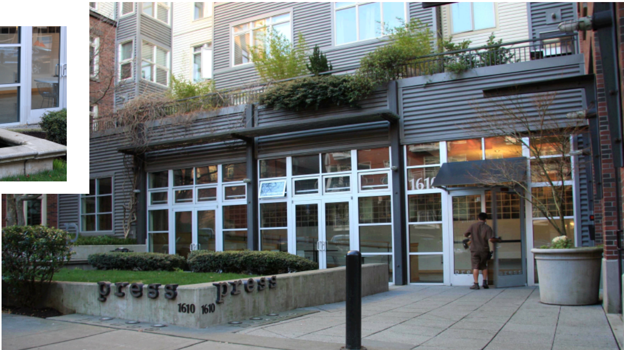
1-STORY COVERED ENTRY WITH 2ND FLOOR GREEN SPACE- COURT YARD HAS SIT WALLS + RAISED PLANTER
