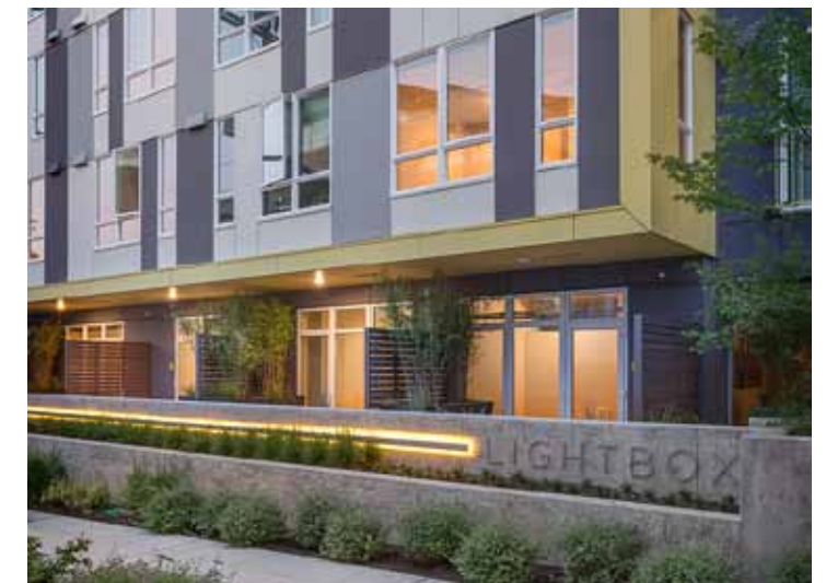
LIGHTBOX - LEED SILVER
