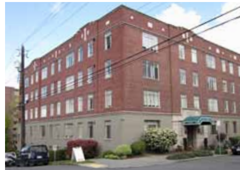
TRADITIONAL BRICK APARTMENT BUILDINGS
