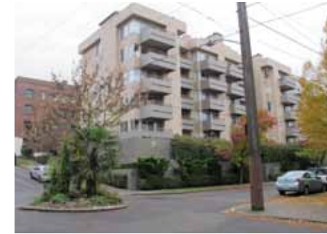
⑦ CASTELLAN APARTMENTS
