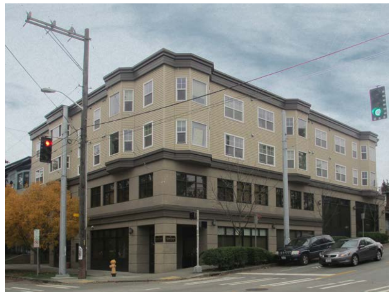
② E Yesler Way and 14th Ave - Bay Windows and Corner Entry
