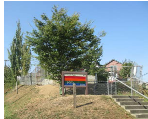
1 Horiuchi Park (under construction)
