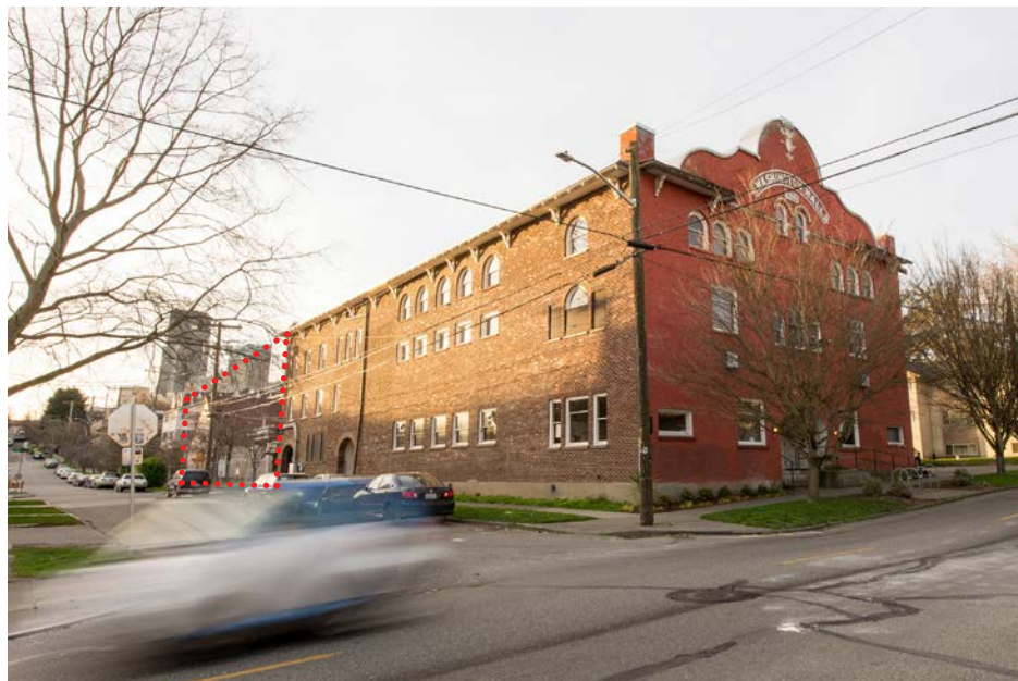
7 View of the site west on E Fir St.
