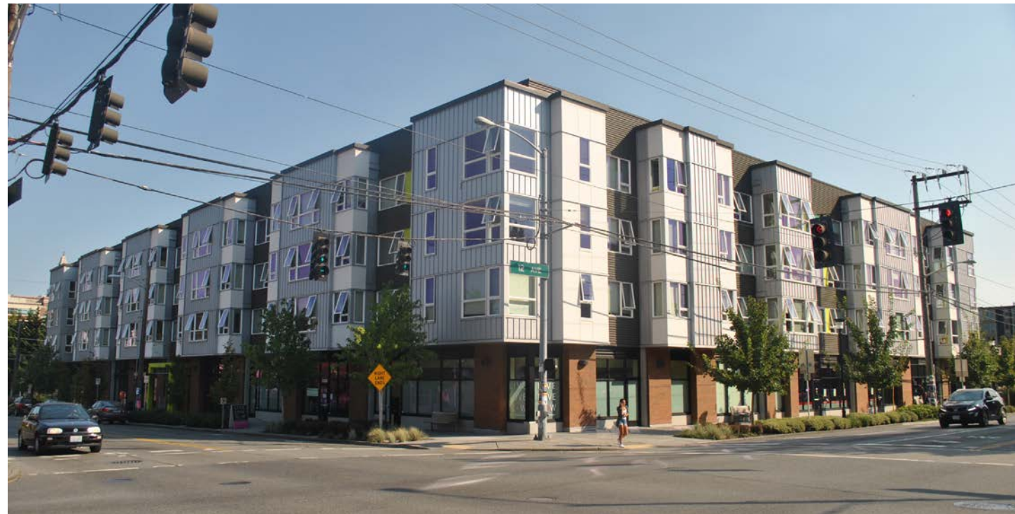
① E Cherry St and 12th Ave - Contemporary Corner Treatment
