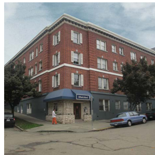
③ E Fir St and 11th Ave - Recessed Corner
