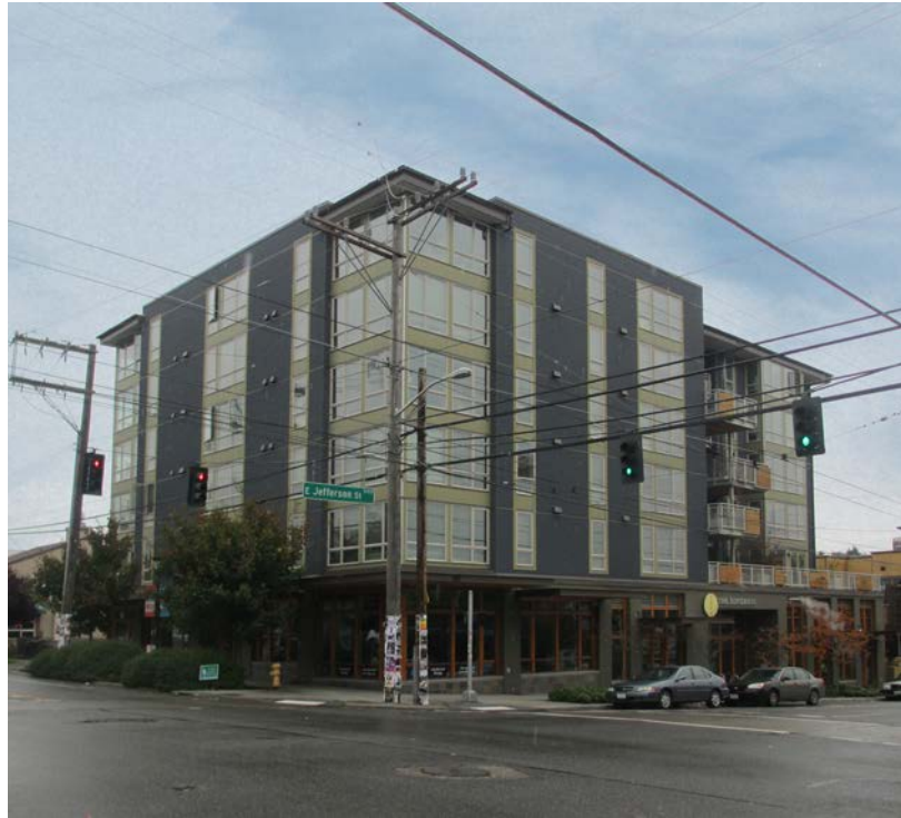
5 E Jefferson St and 12th Ave - Contemporary Materials
