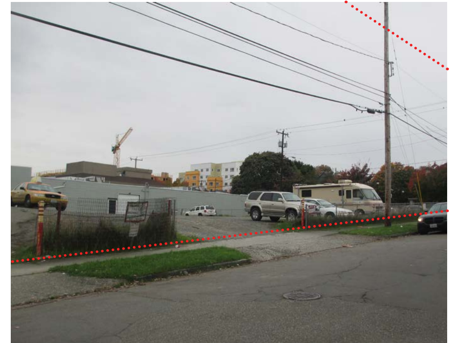
2 View of the site looking southwest on E Spruce street
