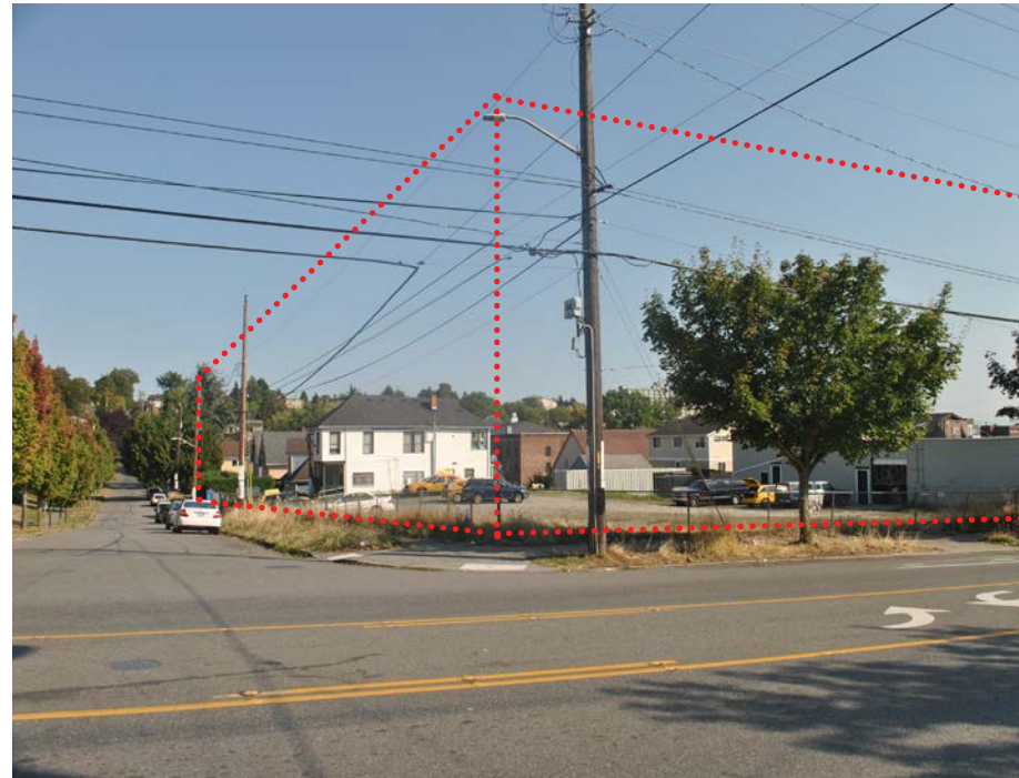
1 View of the site looking southeast on the corner of 12th ave. and E Spruce street
