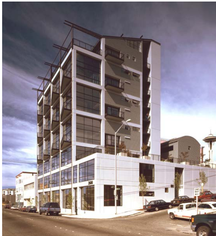
④ Banner Building 74,000 sf Seattle, WA
