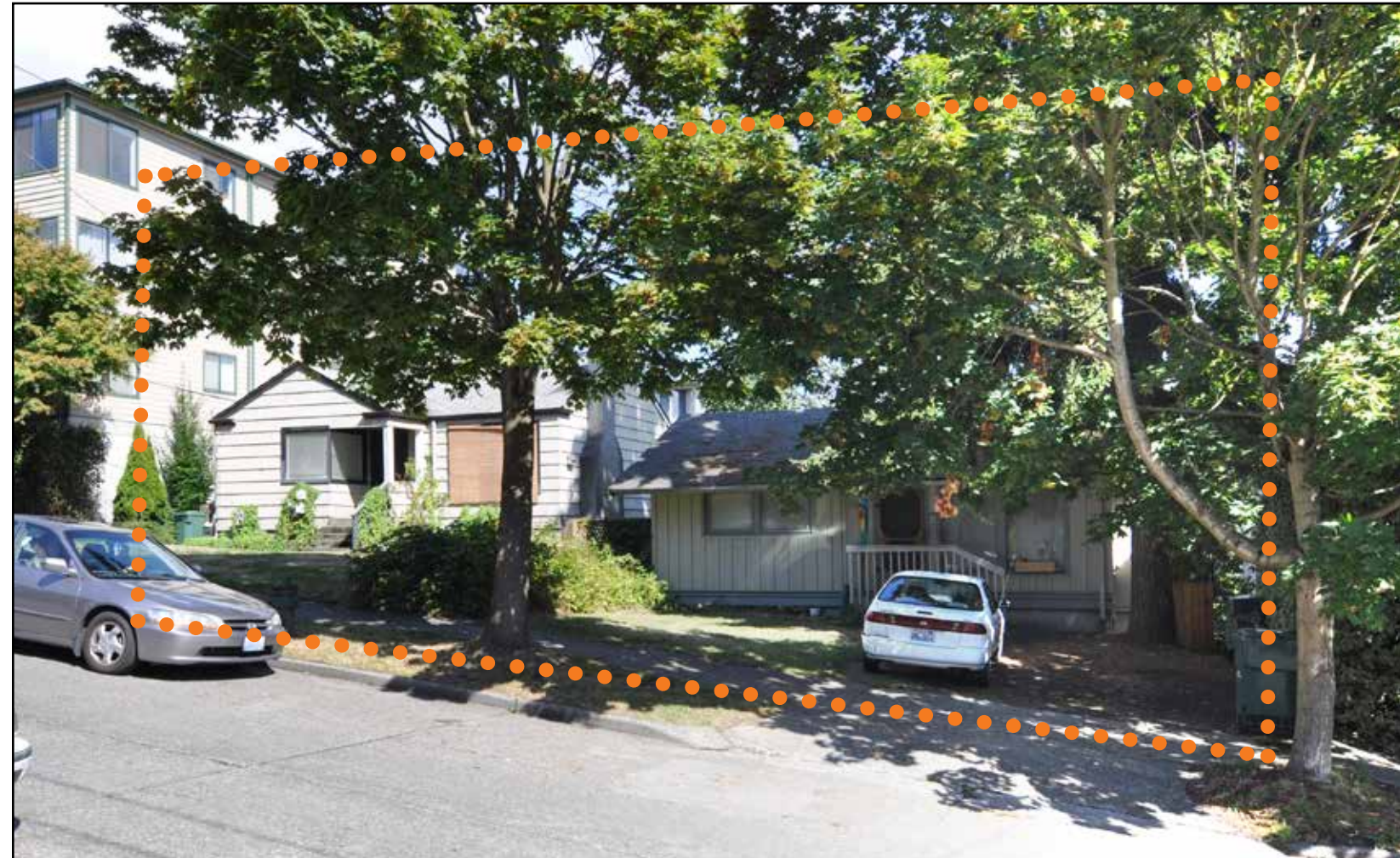
Project Site, existing structures to be deconstructed
