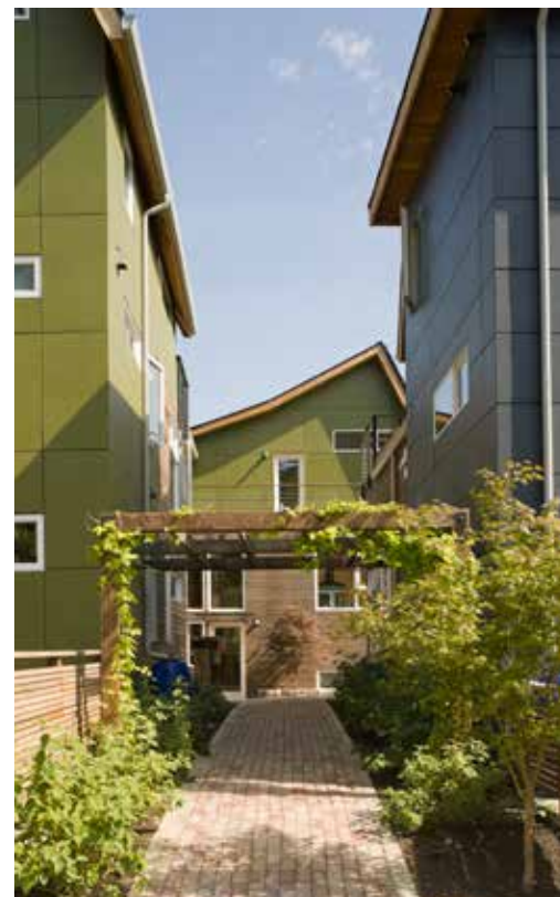
⑤ 1911 E. Pine St. view from street
