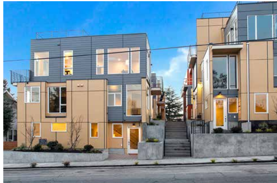
② 3515-19 Wallingford Ave. N. view from street
