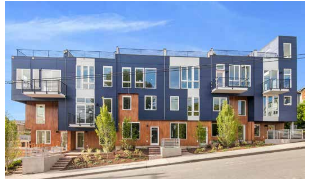
③ 90 E Newton. view from street
