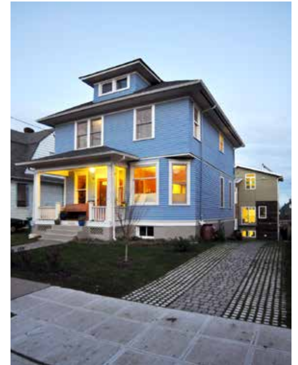
⑧ 1504 19th Avenue Duplex behind SF House
