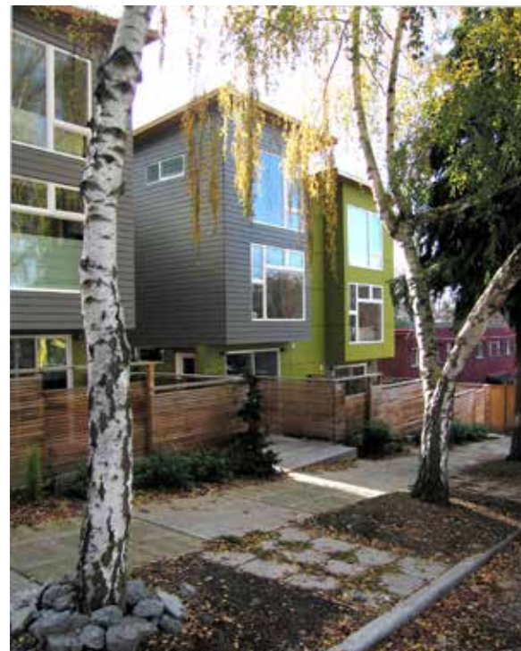
⑥ 1411 E. Fir St. exterior view from street
