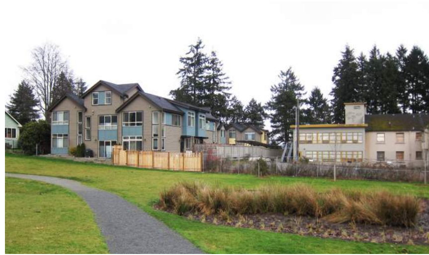
2 EAST VIEW OF SITE
