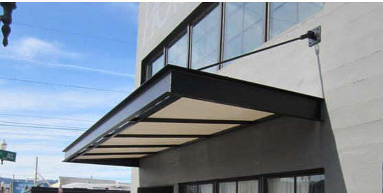
STEEL CANOPY -tall profile, powder coated steel channel with opaque panel and tie rods.
