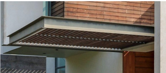
LIVE/WORK CANOPY -shallow profile powder coated steel channel with opaque panel and tie rods.
