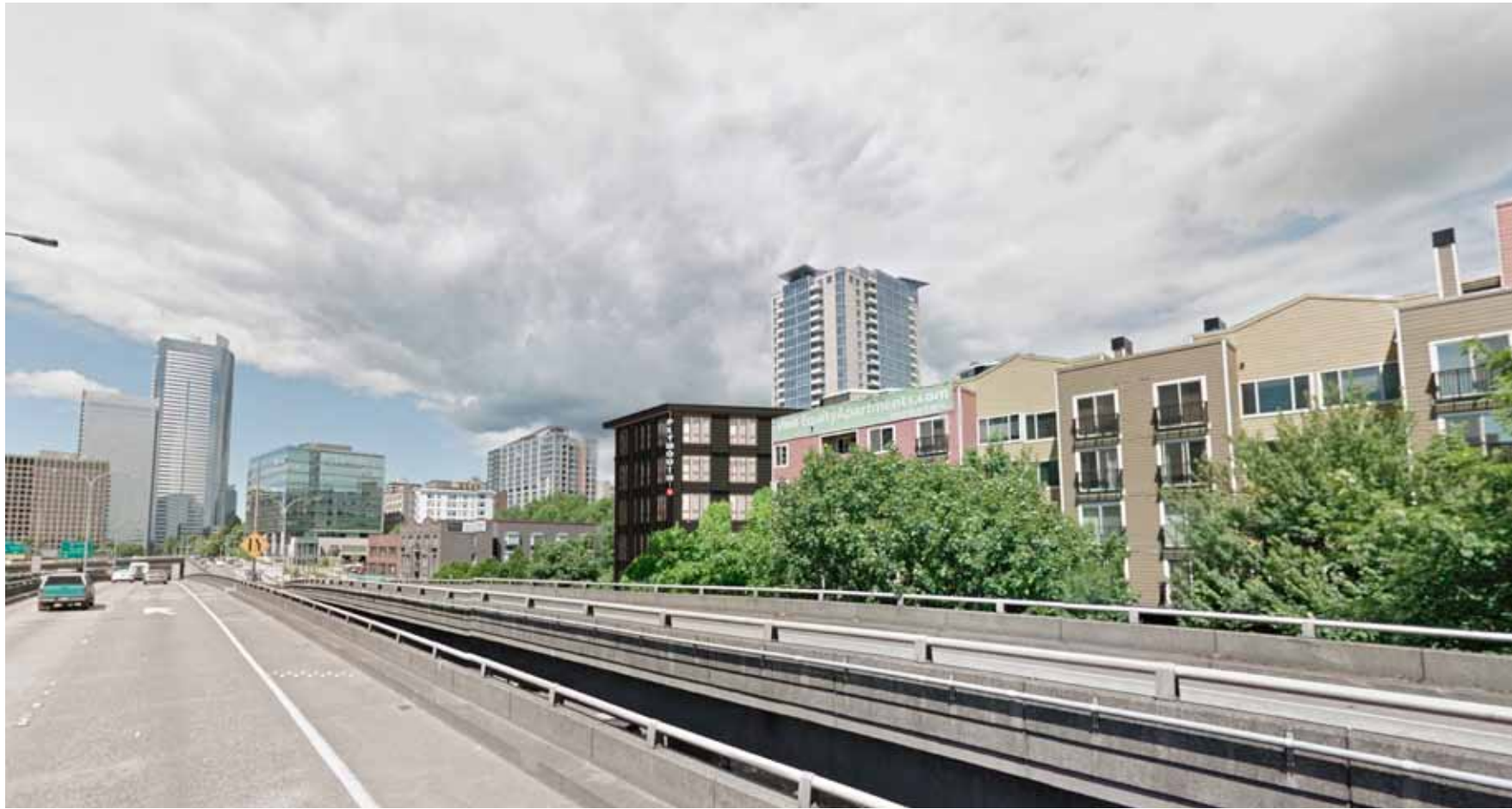
#1 VIEW OF BUILDING FROM I-5 NORTH-BOUND
