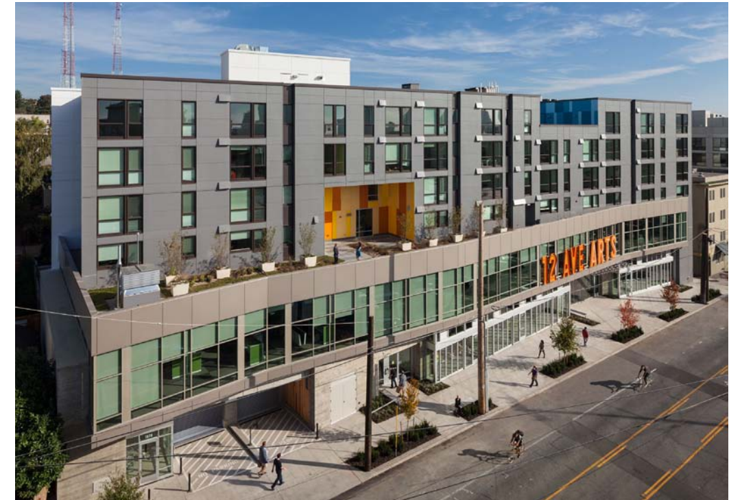
12 Ave Arts 1620 12th Avenue, Seattle, WA Capitol Hill Housing
