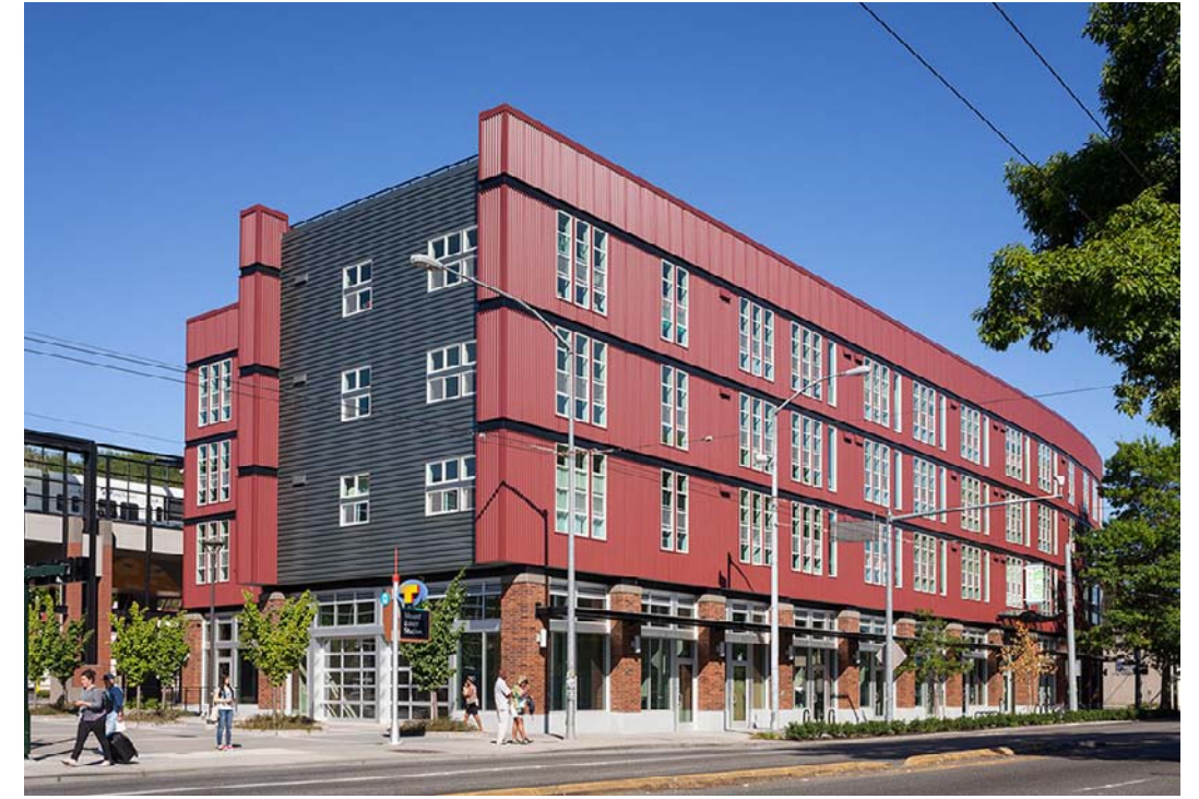
Artspace Mount Baker Lofts 2915 Rainier Avenue S., Seattle, WA, 98144 Artspace Projects, Inc.
