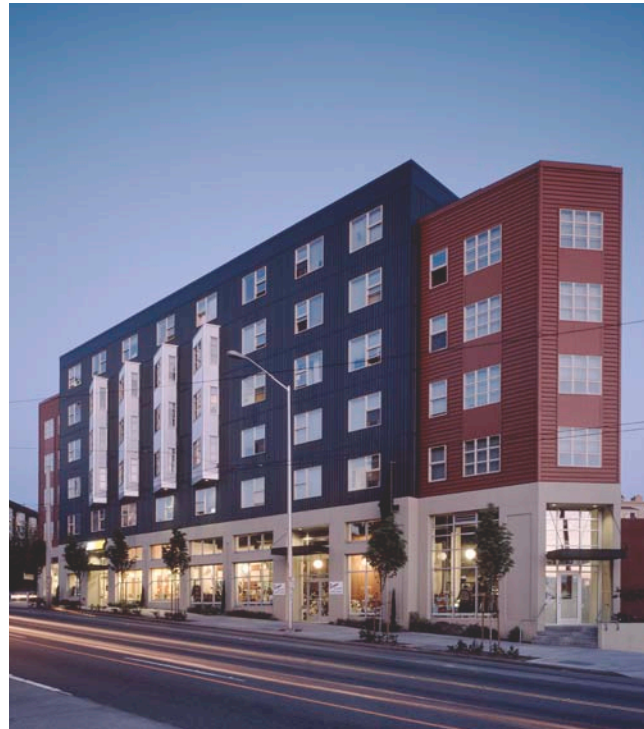
Plymouth Place 94 Bay Street, Seattle, WA Plymouth Housing Group
