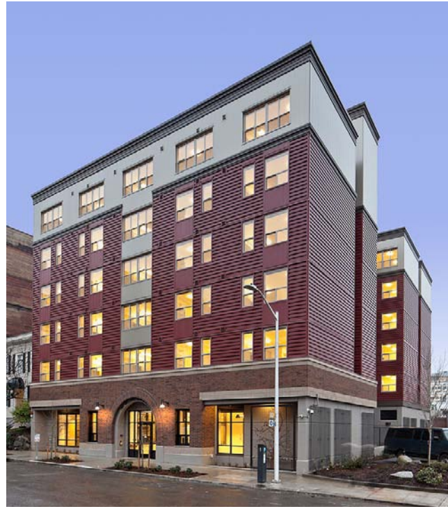
Pat Williams Apartments 219 Pontius Avenue North, Seattle, WA Plymouth Housing Group
