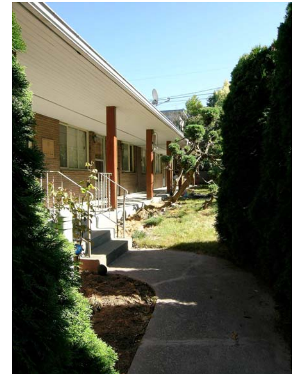
2. EXISTING APARTMENT FROM S
