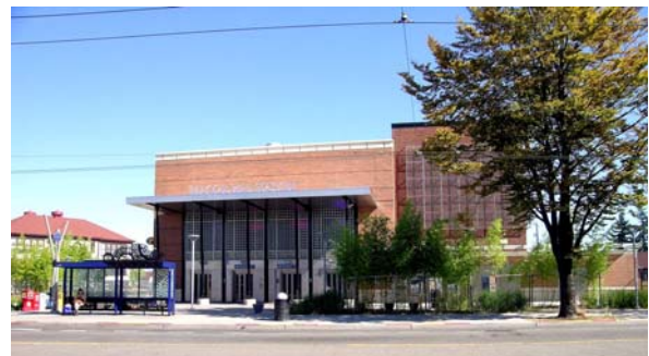
LINK LIGHT RAIL STATION
