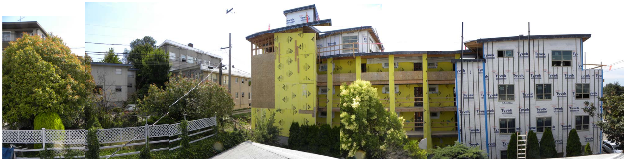
5. LOOKING EAST AND SOUTH FROM SITE
