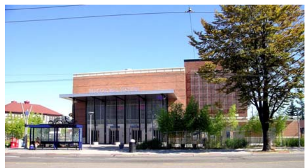
LINK LIGHT RAIL STATION
