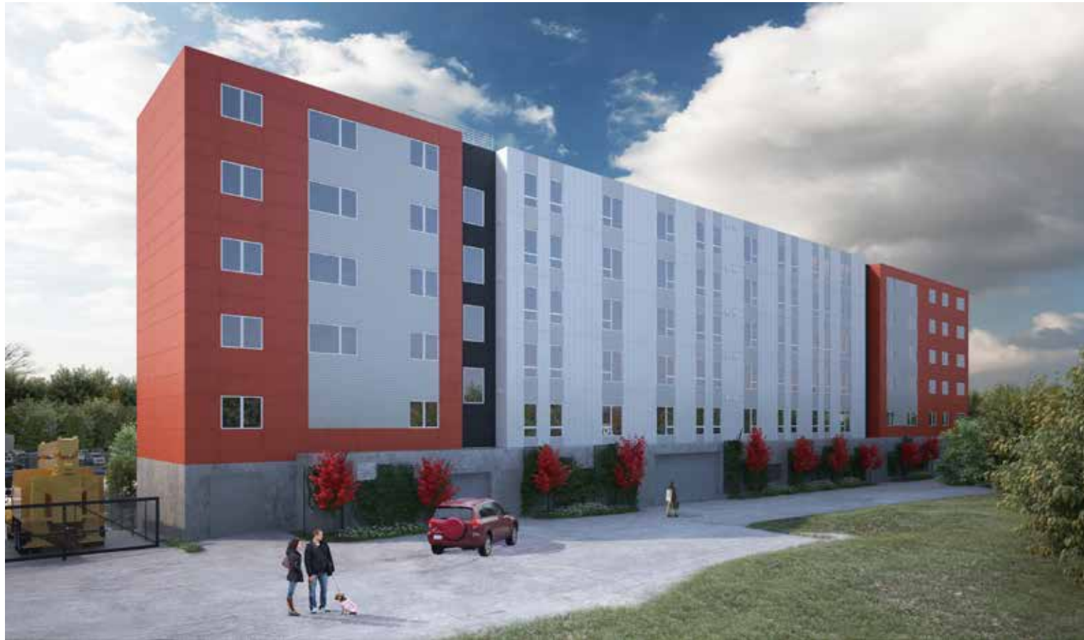
VIEW OF EAST FACADE 7.14.15
