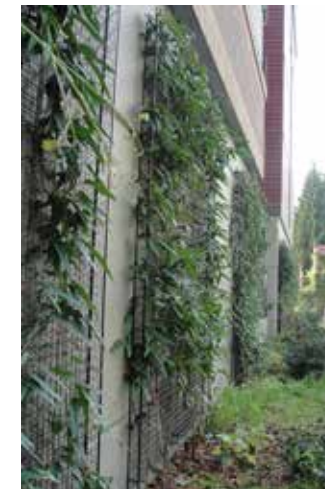
BLACK GREENSCREEN PANELS WITH CLIMBING VINES
