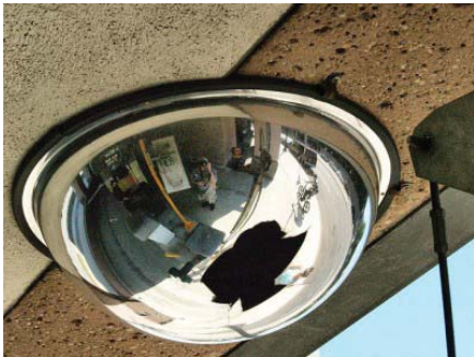
1. Domed Mirror Installed above entry to ensure full visibility from all angles
