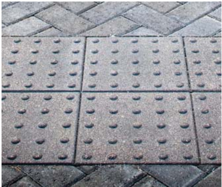
2. Truncated Dome Tactile Warning Located @ each end of garage entry to provide warning for the visually impaired
