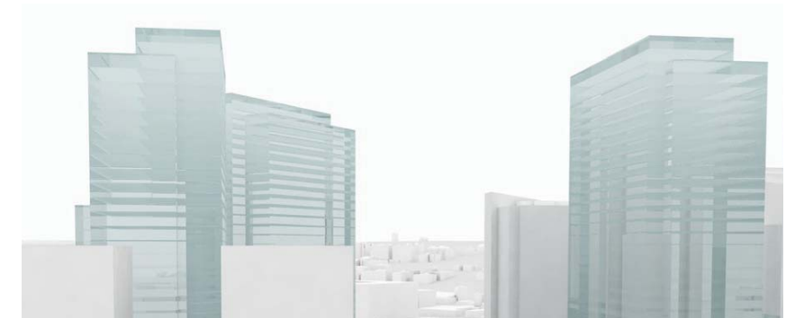
11. Amazon Towers (Under construction)
