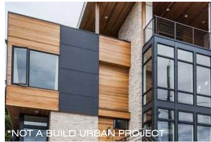
Black windows as material upgrade
