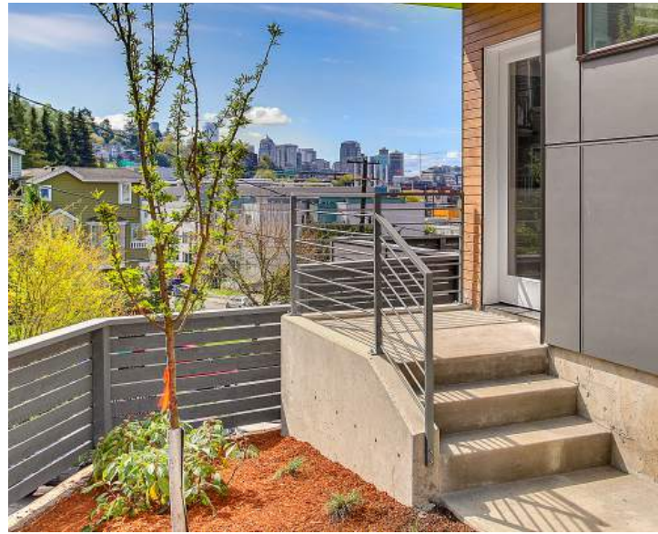
Natural concrete stoop and dark gray powder coated metal railing
