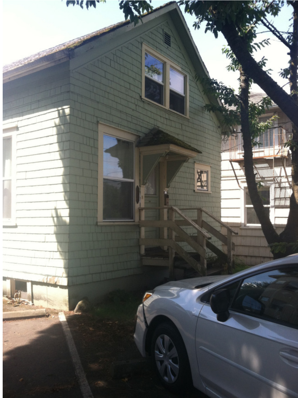
EXISTING HOME TO BE DEMOLISHED
