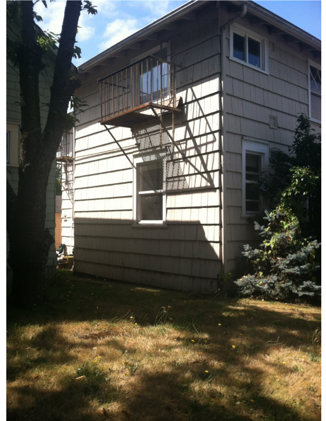
EAST ELEVATION OF EXISTING NEIGHBOR TO THE WEST
