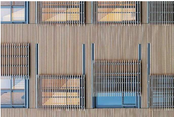
Operable screening blends with the facade while introducing an element of chaos and randomness to the building.
