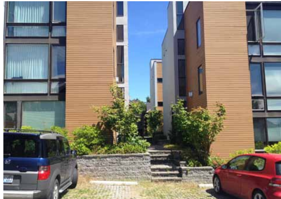
2. Density of properties and utilization of alley. Layering of textures and materials.
