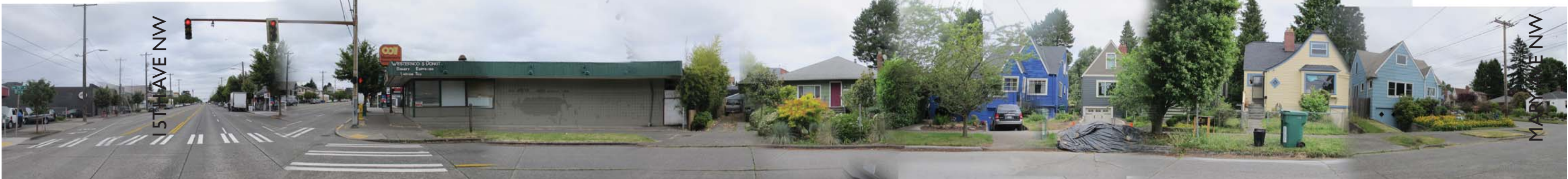
④ NW 75TH ST LOOKING NORTH
