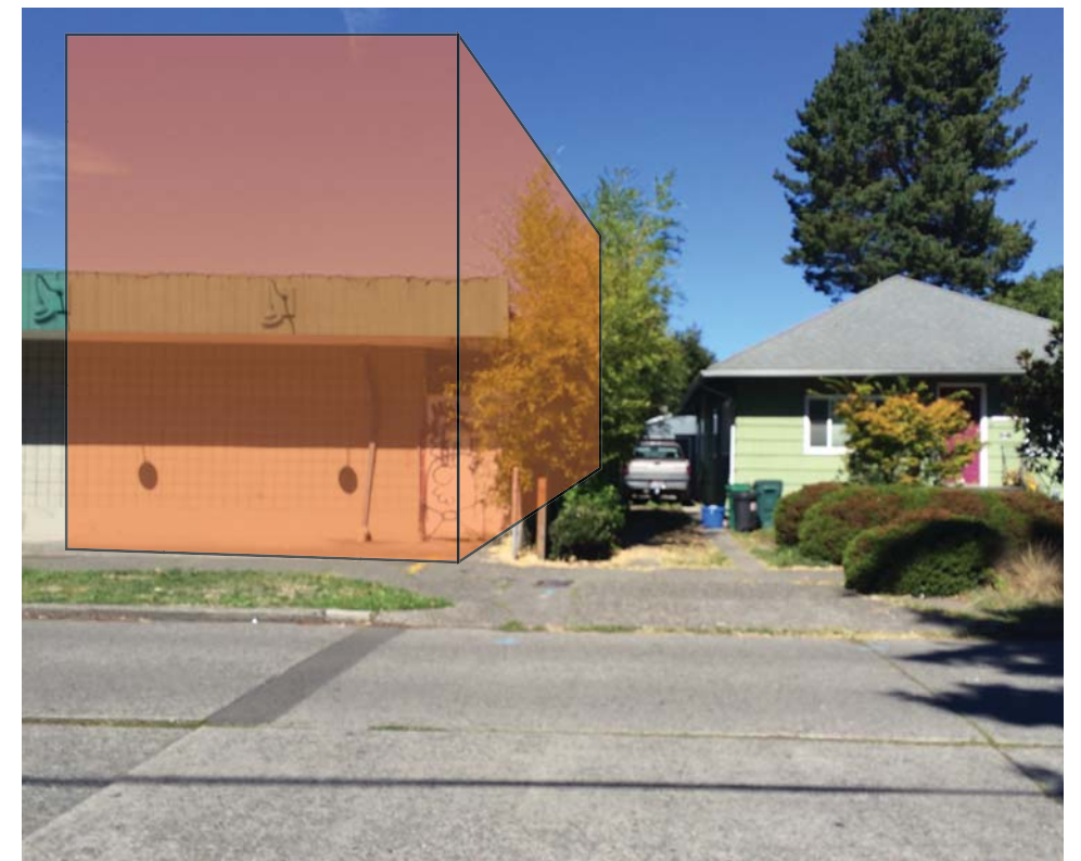
⑩ VIEW OF SOUTH PROPERTY LINE AND NEIGHBORING HOUSE
