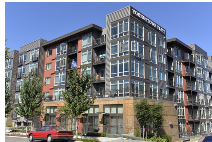
4040 26th Avenue SW - Youngstown Flats
