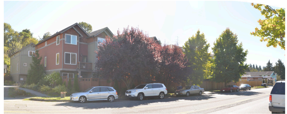
Project Site - 5206 Delridge Way SW from SW corner of Puget Blvd. SW and Delridge looking southeast
