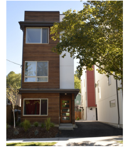
4146 25th Avenue SW
