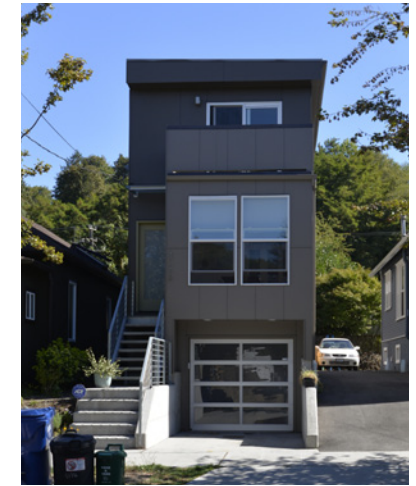
4106 25th Avenue SW
