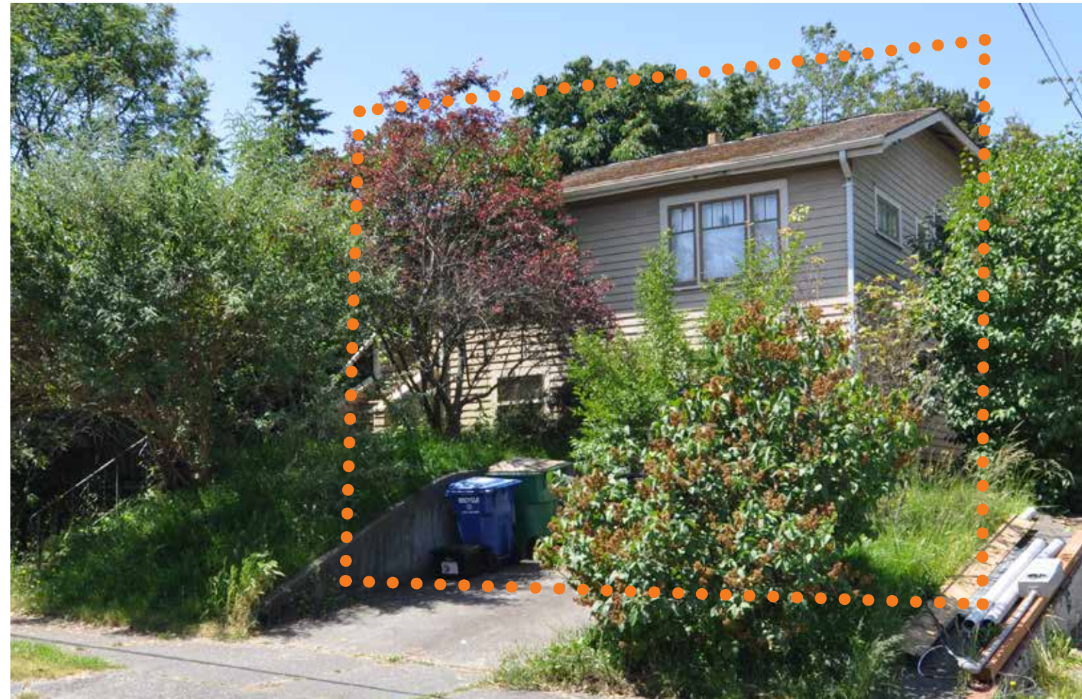
Project Site, existing single family structure to be deconstructed.
