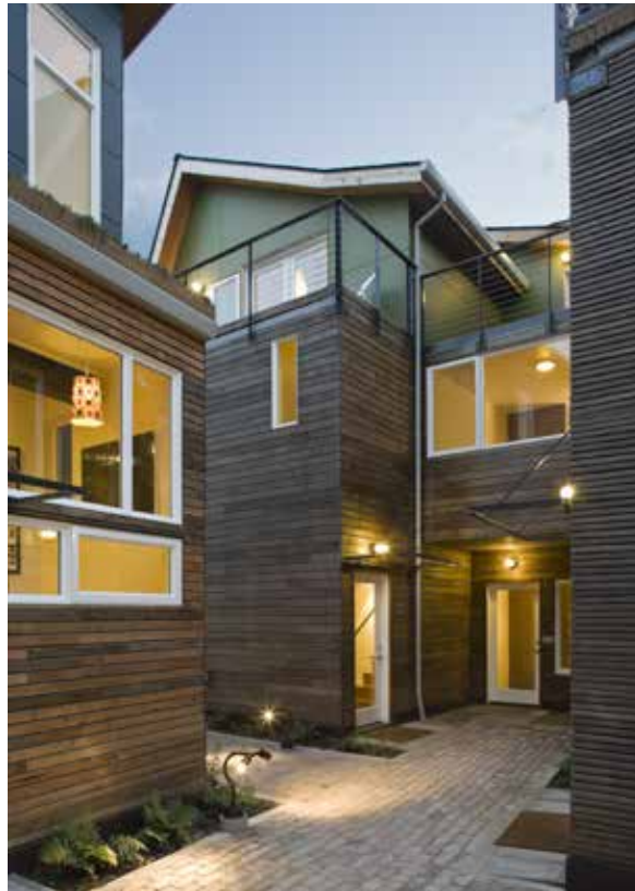
⑤ 1911 E Pine St. view at interior of canyon
