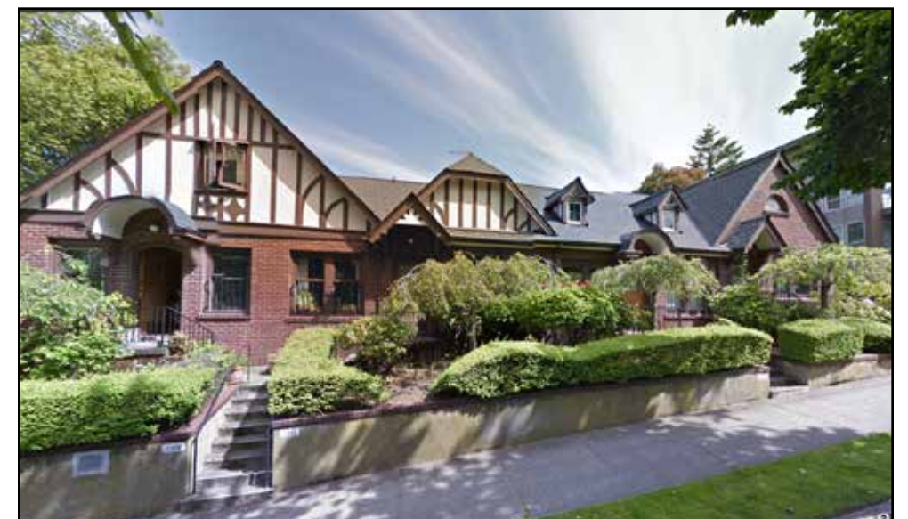
② 1300 E Mercer Apartment Built: 1926
