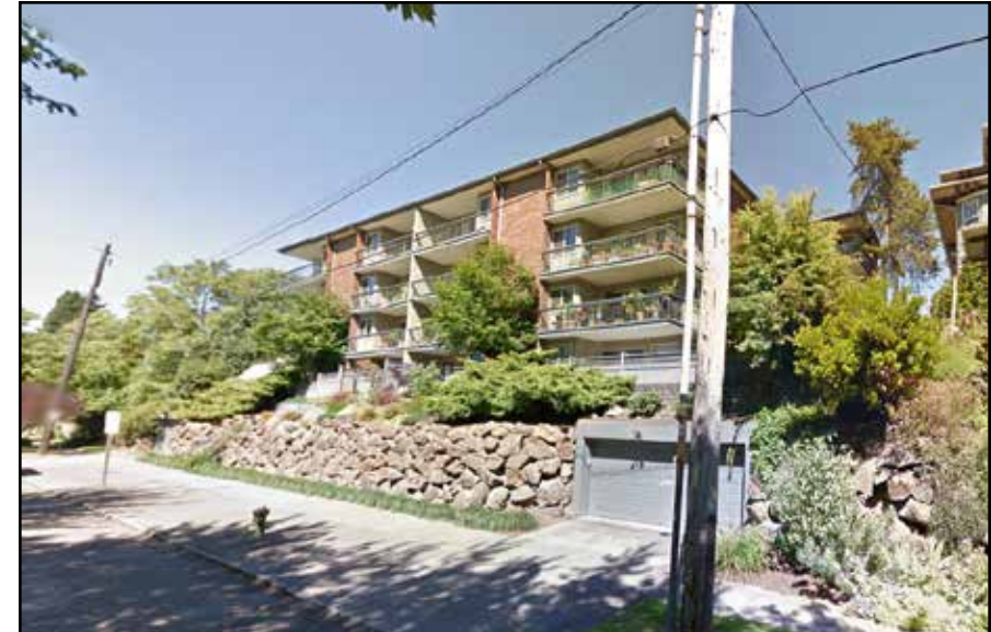
5 Midtown Condominiums Built: 1969
