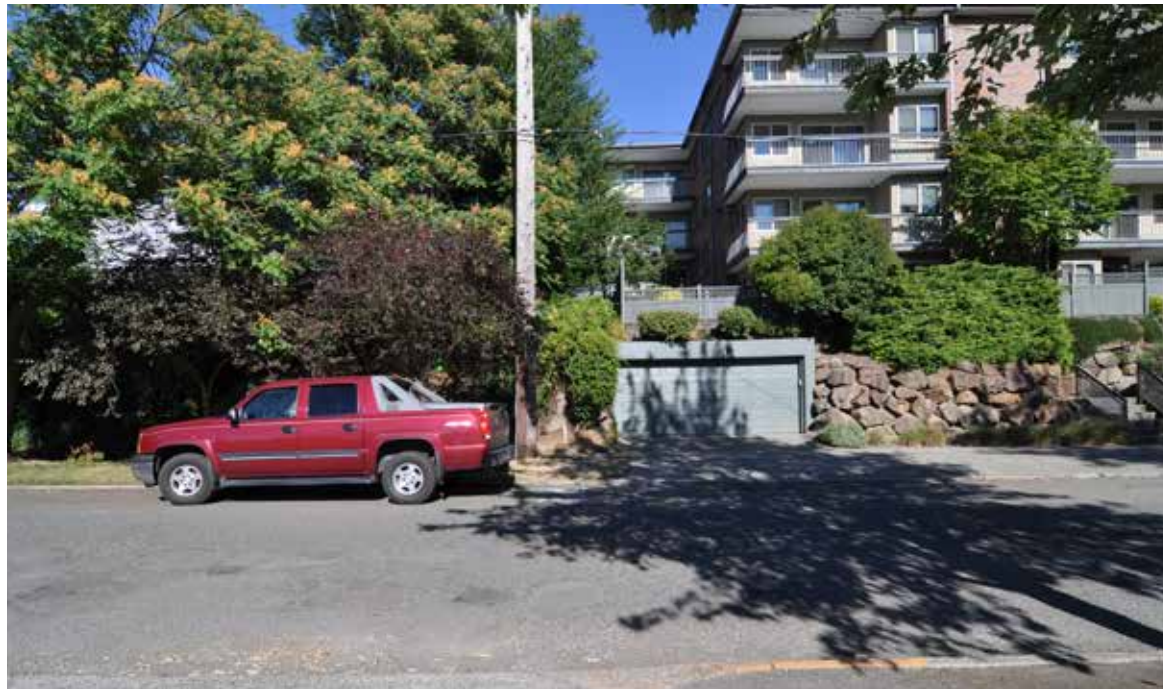
1 Property Line from 11th Avenue E Looking E
