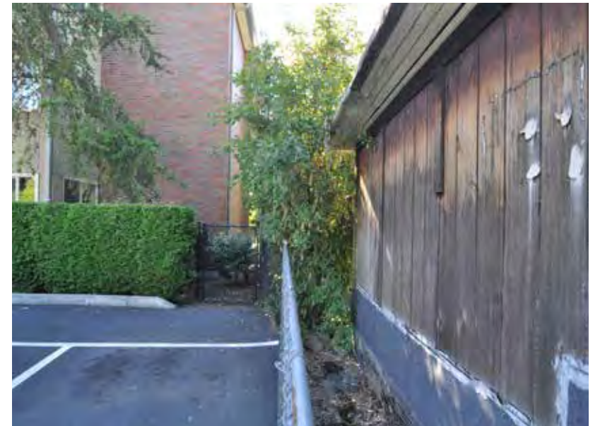
2 Property Line from Alley Looking W
