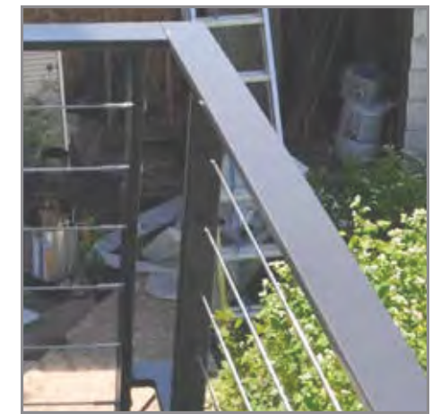
Steel Exterior Railing
