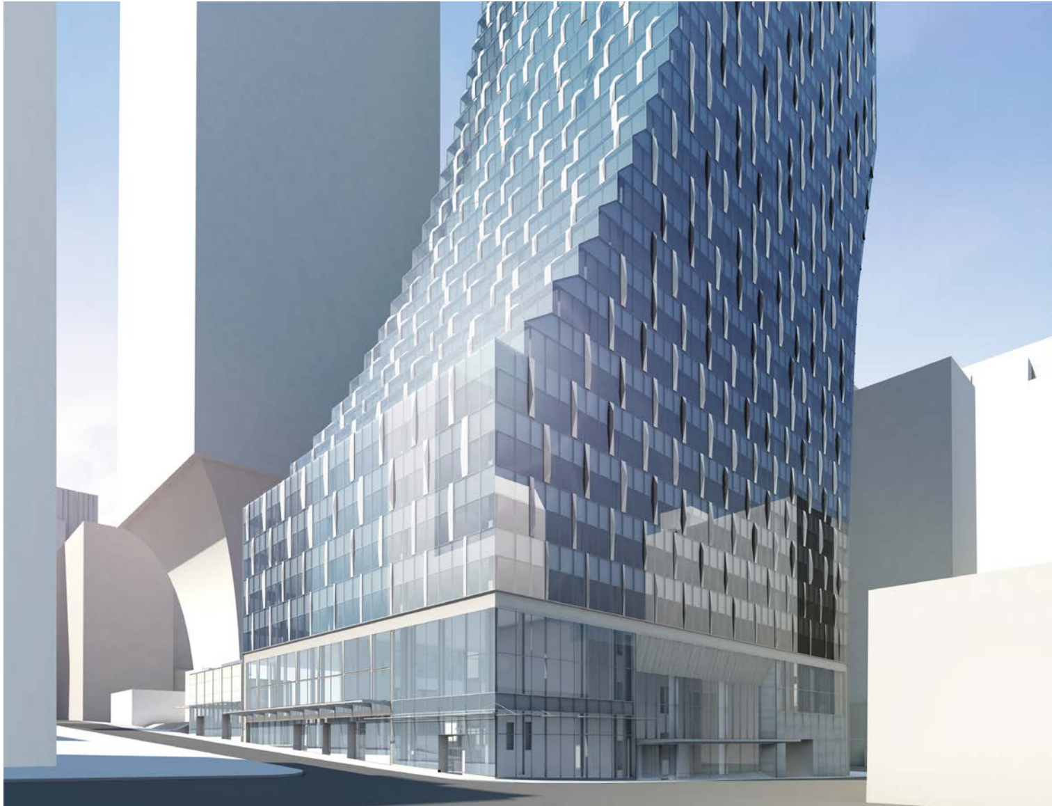
Street level view looking southwest - Level 7 datum
