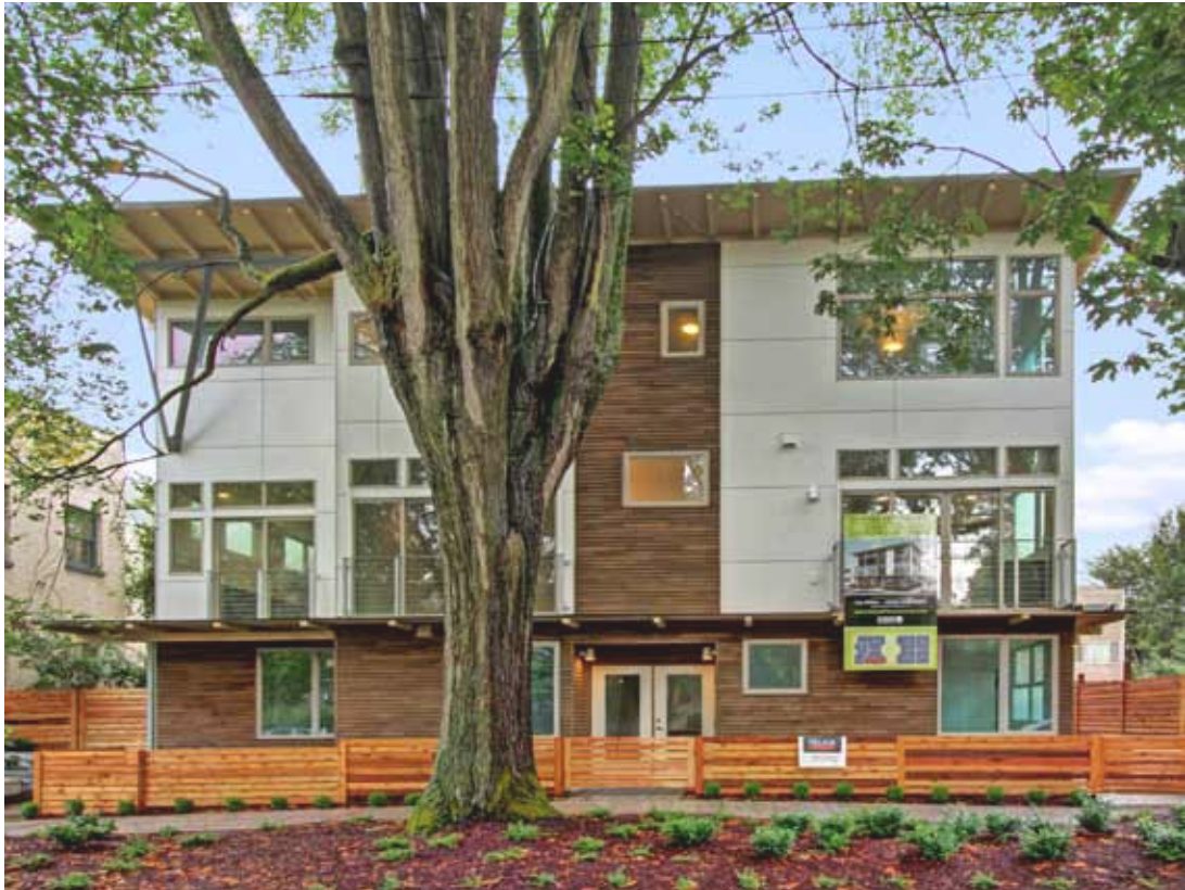
ROOF OVERHANGS AND EXPOSED TIMBER FRAMING CREATE AN EXPRESSIVE AND DETAILED BUILDING TOP (1724 17TH AVENUE)
