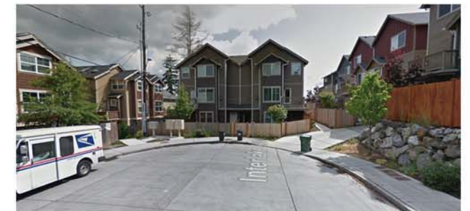
E - LR3 - Recent Townhome development. The multifamily developments throughout Licton-Springs have increased residential density in the last ten years but primarily with townhomes. An apartment building with a variety of units from studio to three bedrooms would provide more diversity to the housing market.
