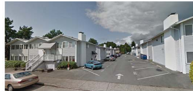
B - LR2 - Apartment complex - Many existing multifamily structures have dedicated onsite parking. Although the project is not required to provide parking by City code parking may be necessary to compete with similar rentals throughout the neighborhood. Parking should be located from the alley and below grade to preserve all street front commercial opportunities.
