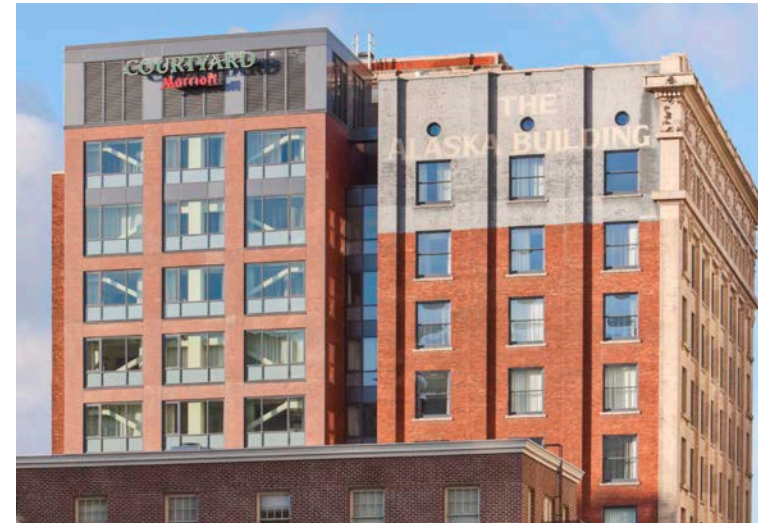
Alaska Building - Hotel Renovation/Addition (Complete 2009)
