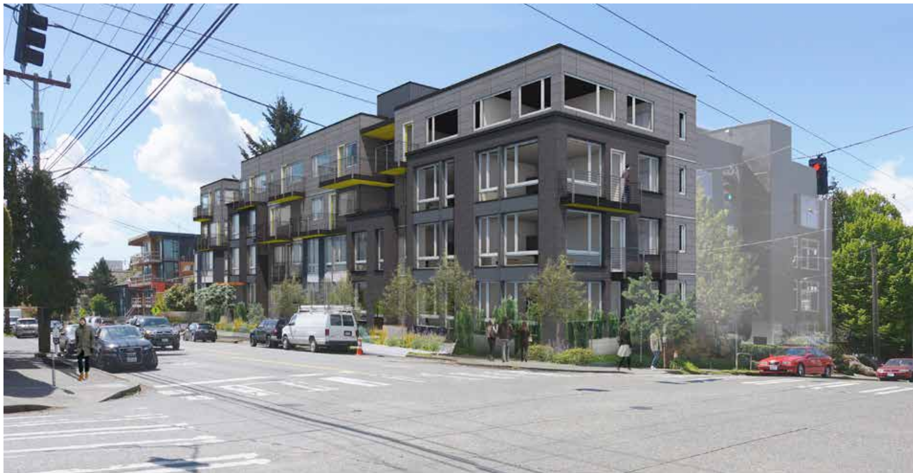
View from NE
