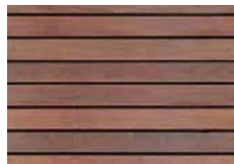
Gapped Hardwood Siding
