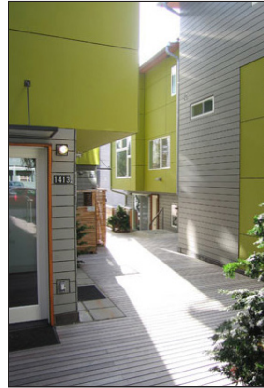
1411 E. Fir St. courtyard view
