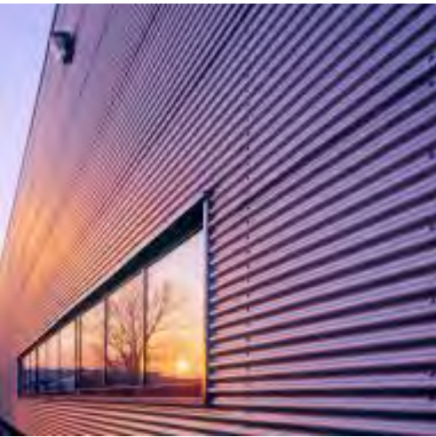
CORRUGATED METAL SIDING (LOCATED ON EAST BUILDING)
