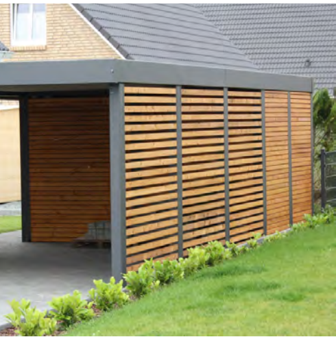
PAINTED WOOD CARPORT WITH CEDAR AND METAL SCREENING (LOCATED AT CENTRAL PLAZA)
