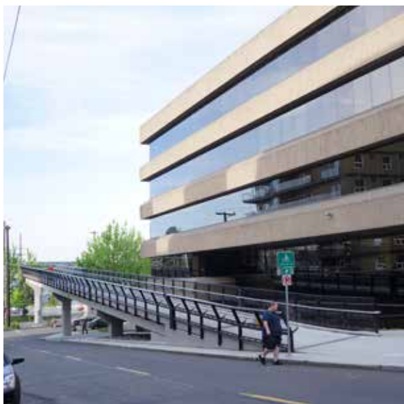
M Elliott Bay Office Park + Thomas St. Overpass
