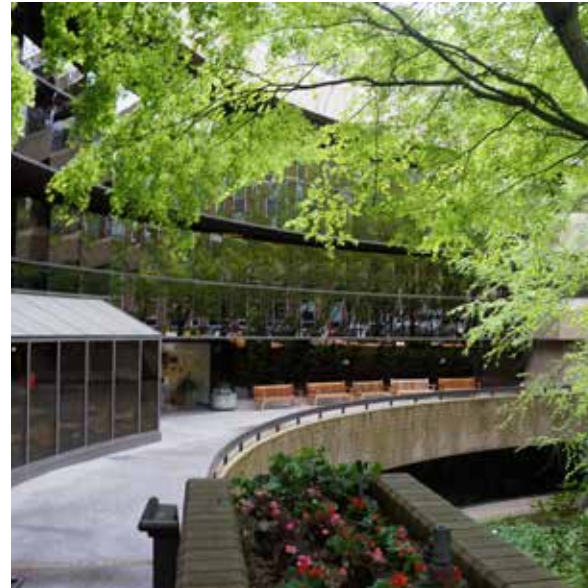
C Entry Court at Elliott Bay Office Park
