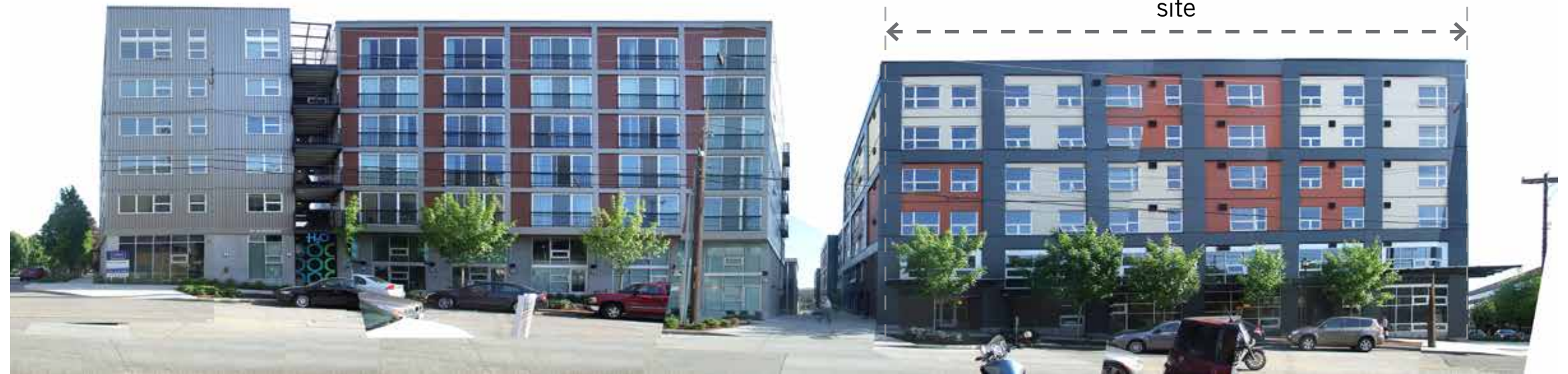
1a W Harrison St. from Site
