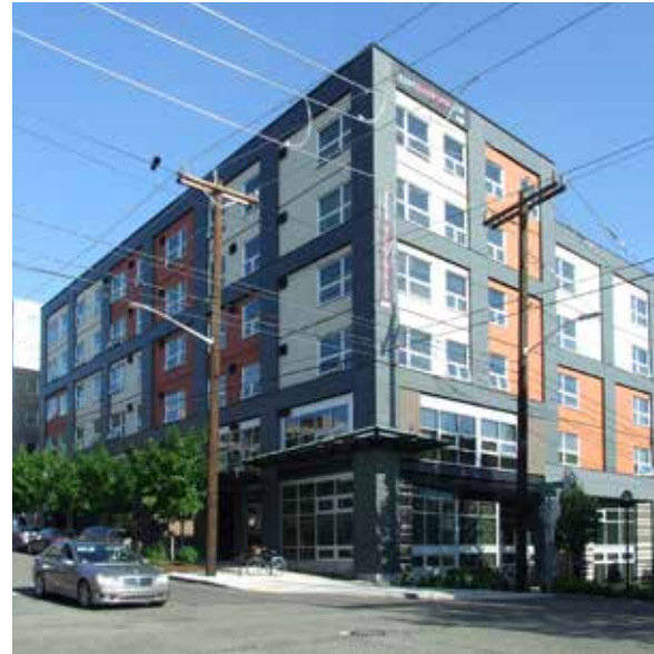
D Avalon Bay Apartments (Harrison St)
