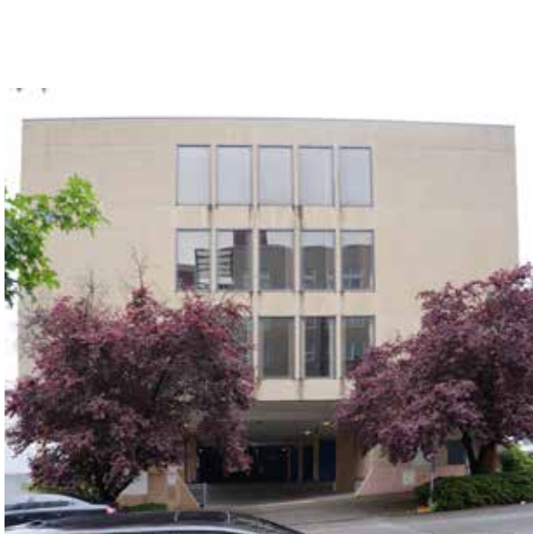
F Office Building at 2nd Ave + Harrison St
