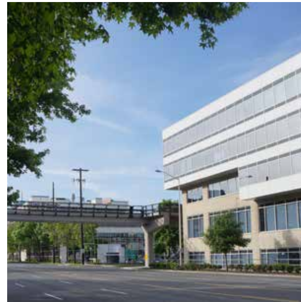
I 333 Elliott + Thomas St Overpass
