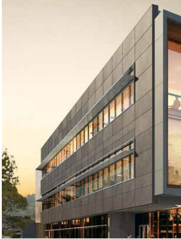
Linear windows and solar shades
