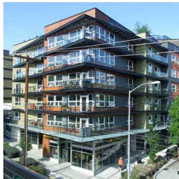
N Avalon Bay Apartments (Thomas St)
