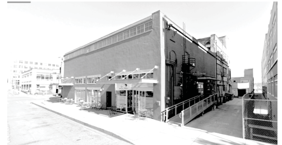
C. REPUBLICAN ST. AT ALLEY LOOKING INTO SITE
