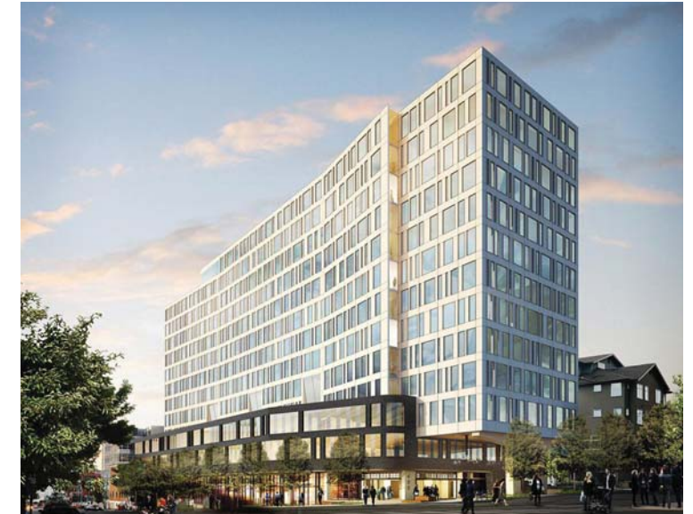
400 Fairview (In Construction) H
