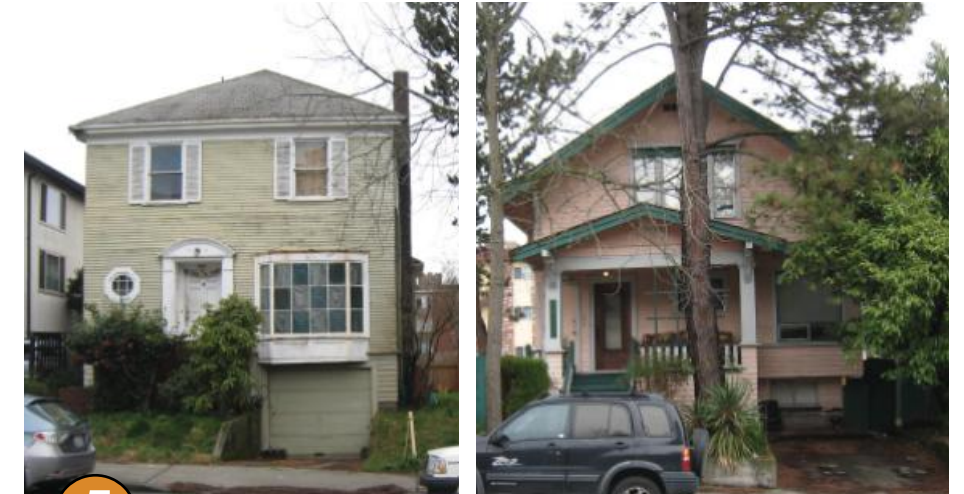
5 single family residences on site
