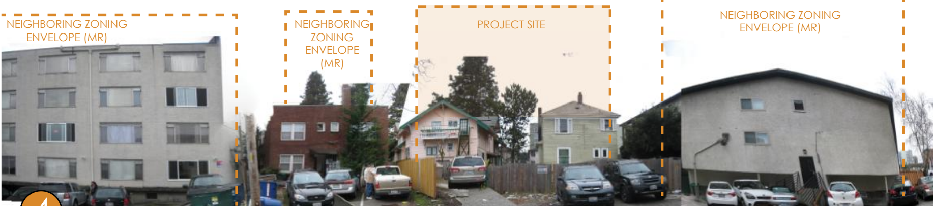
4 Alley, looking W at project site
