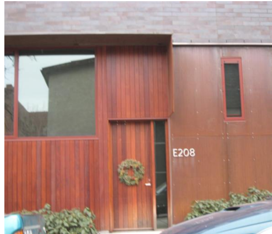
Variety of materials used in building palette
