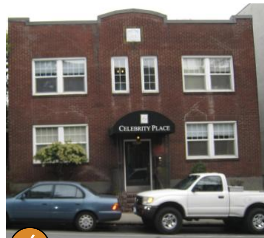
6 two story apts S of site on 11th Ave NE
