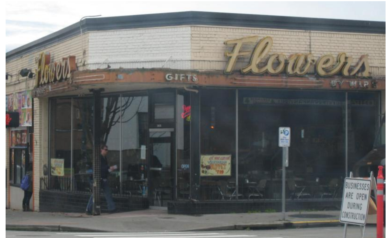
Large pedestrian-oriented storefront windows; durable building materials
