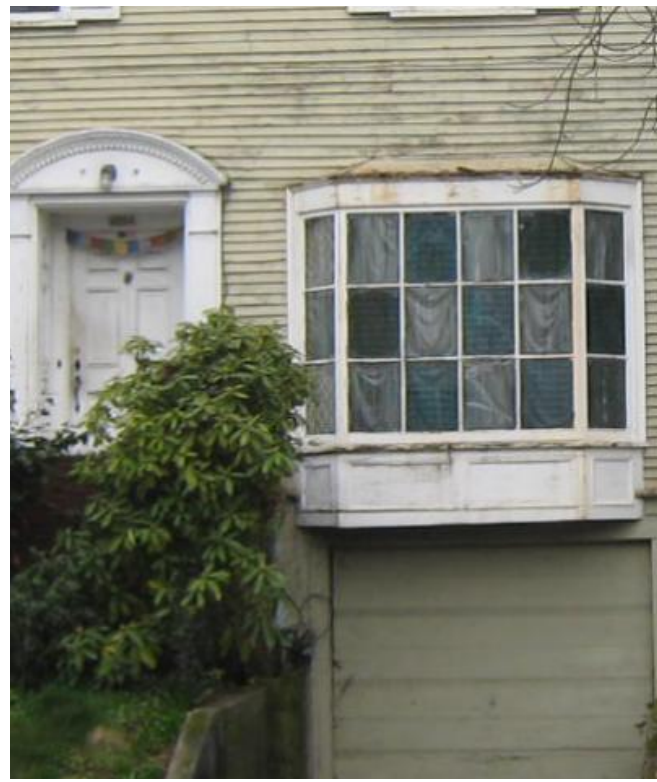
Bay window at existing building
