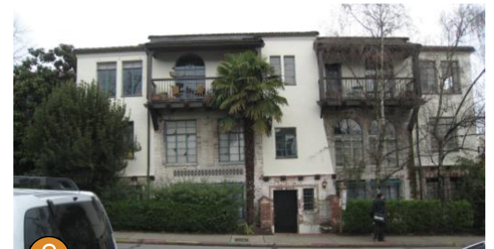
8 three story apts S of site on 11th Ave NE
