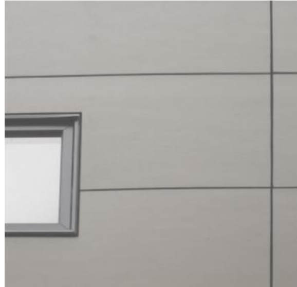
Painted cement board panel siding
