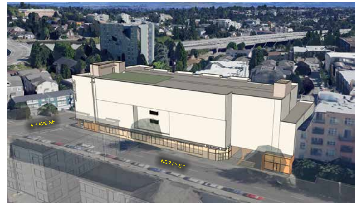
AERIAL VIEW NORTHWEST
