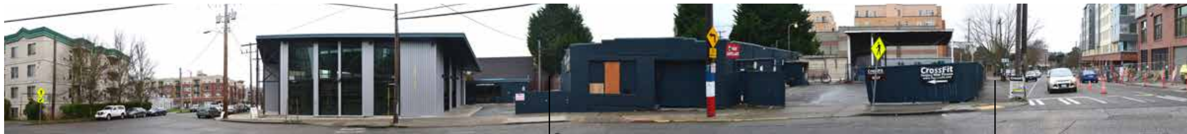
③ 5 TH AVENUE NE LOOKING WEST TOWARD PROJECT SITE
