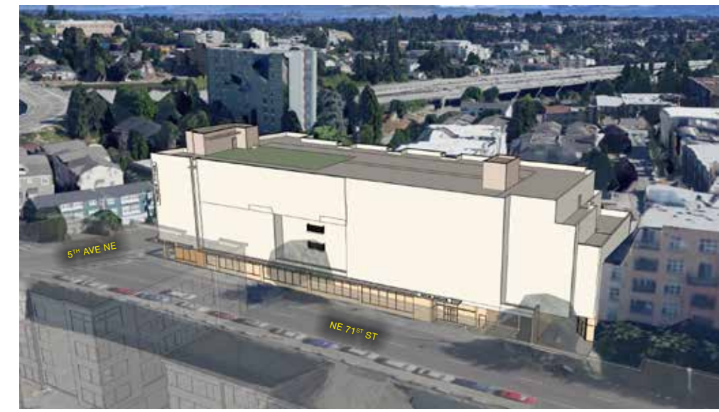
AERIAL VIEW NORTHWEST
