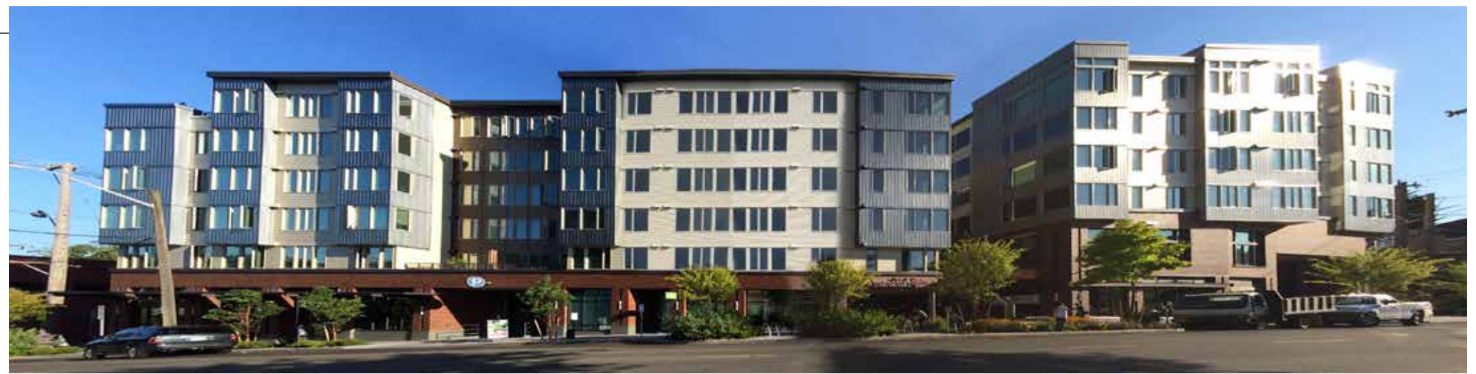
① NE 71 ST STREET LOOKING NORTH
