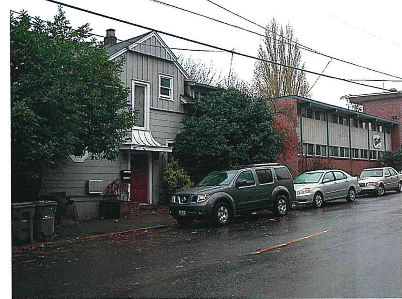
6 Rooming house and apartment south of 4714
