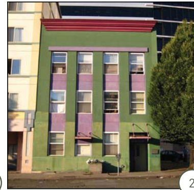
ARION COURT APARTMENTS 3 Floors - Apartments 1814 Minor Avenue
