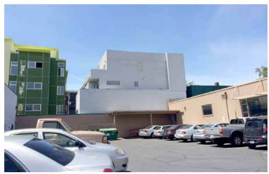
EXISTING APARTMENTS TO WEST OF SITE
