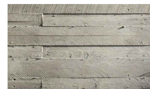
EXPOSED BOARD FORMED CONCRETE
