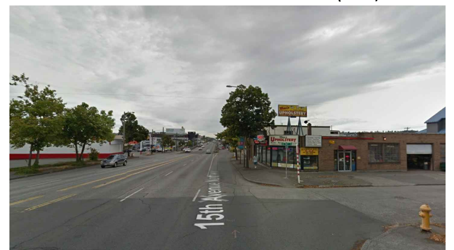
15TH AVE NW - LOOKING SOUTH (beyond site)
