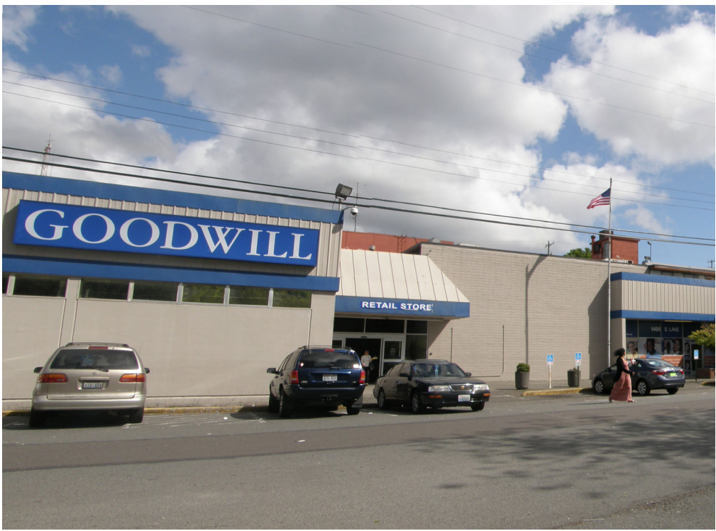
A GOODWILL JOB TRAINING AND EDUCATION CENTER
