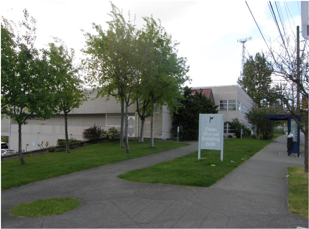
C PEARL WARREN BUILDING
