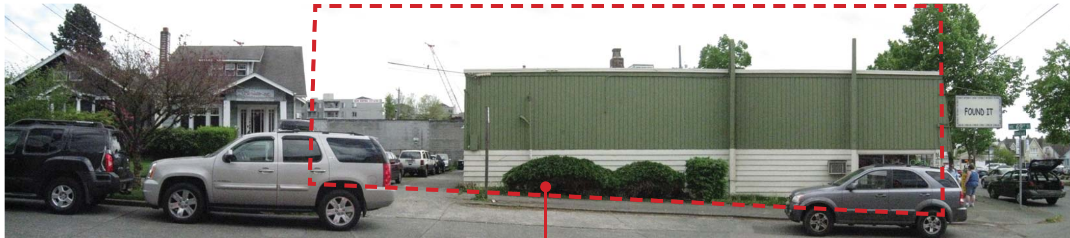
③ NE 69th Street - South Side
