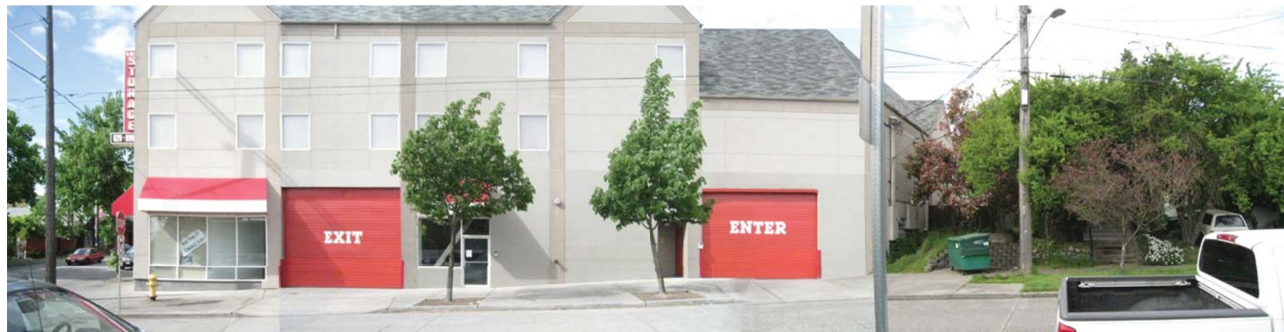
③ NE 69th Street - North Side
